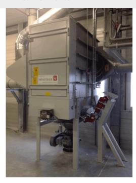
For dedusting the manufacturing process of special chemicals an **aspiration filter of type Infa- Lamellen-Jet** is used. In spite of small floor space a filter surface of 72 m<sup>2</sup> could be realised because of the optimised filter geometry.
