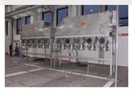
Dedusting of two stainless steel caissons, in which radioactive waste is disaggregated, sorted and reconditioned, is carried out by two identical **cassette filters**, **type INFA-MICRON MKR 5/20-4/20**. The cassette filters were planned with two filter stages in order to achieve a higher cleaning efficiency of the slightly nuclear dust.
