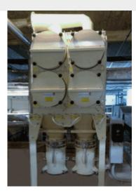
A **cartridge filter type INFA-MICRON MPR 2/20-2/20** cares for a clean production of pharmaceutical products by gathering the dust at several suction points from a tablet press.
